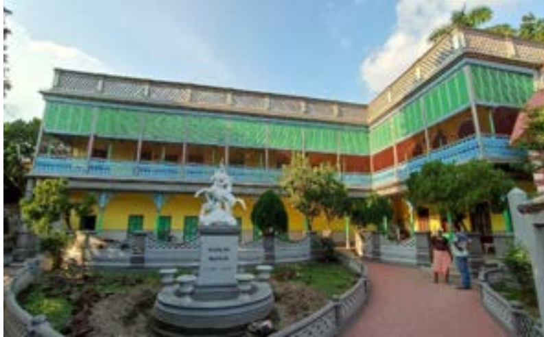
A common typology of residential mansions evolved during 20 th century with cast-iron ornamental railings and wooden Jhillis/screens
