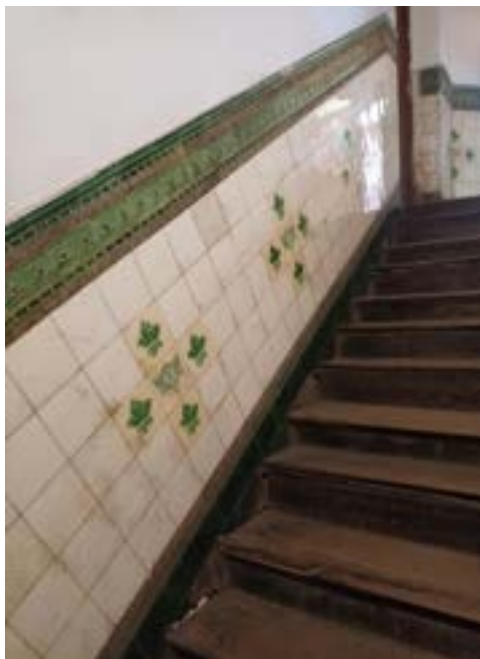
wooden staircase with glazed dado(original)
