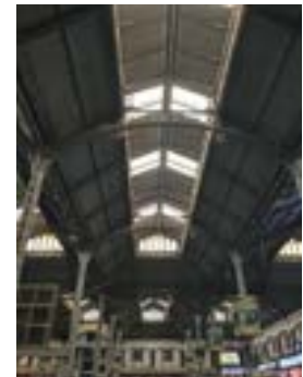
use of transparent sheet on roof for the natural light
