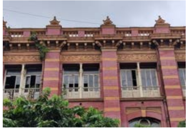
ornamental features with Bands on red exposed brick construction
