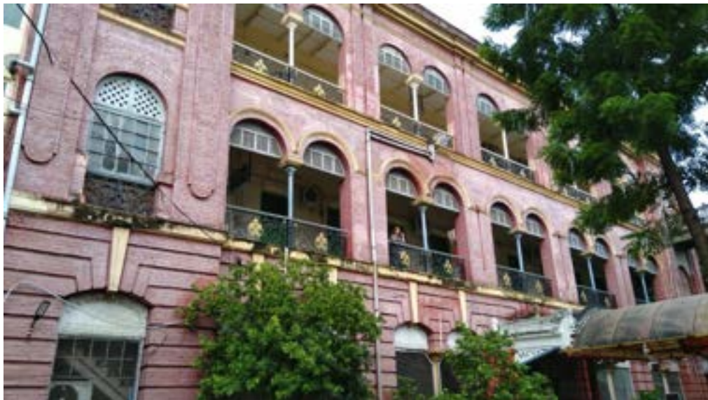
Arched veranda with C.I ornamental Grill and rusticated exposed brick walls at ground floor
